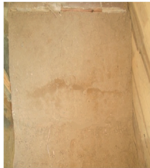
(a) Sand embankment slope without failure
